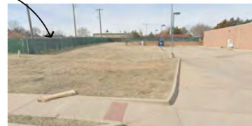
2 EXISTING CONDITIONS IMAGE
