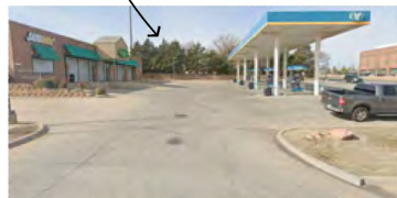
1 EXISTING CONDITIONS IMAGE
