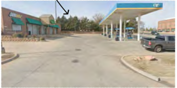
1 EXISTING CONDITIONS IMAGE
