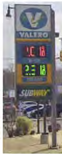
EXISTING DF SIGNS TO BE REFACED WITH NEW FACES. ALL EXISTING CABINETS, RETAINERS & POLE TO BE REPAINTED TRICORN BLACK.
