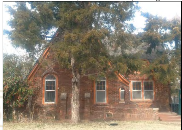
829 NE 16 th Street, South Elevation, Existing
