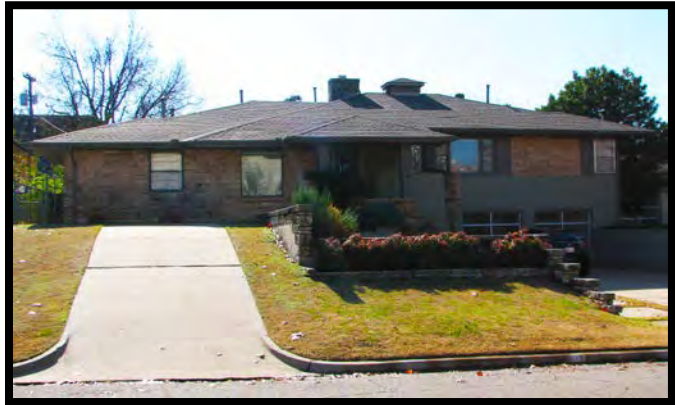
FIGURE 18: EXAMPLE OF THE RANCH STYLE, 608 N.E. 19TH ST.
