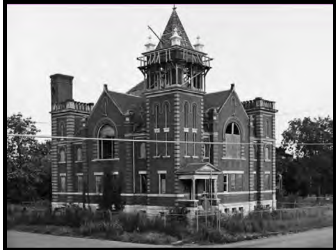
FIGURE 6: THE MAYWOOD PRESBYTERIAN CHURCH BEFORE REHABILITATION IN THE 1980S.
