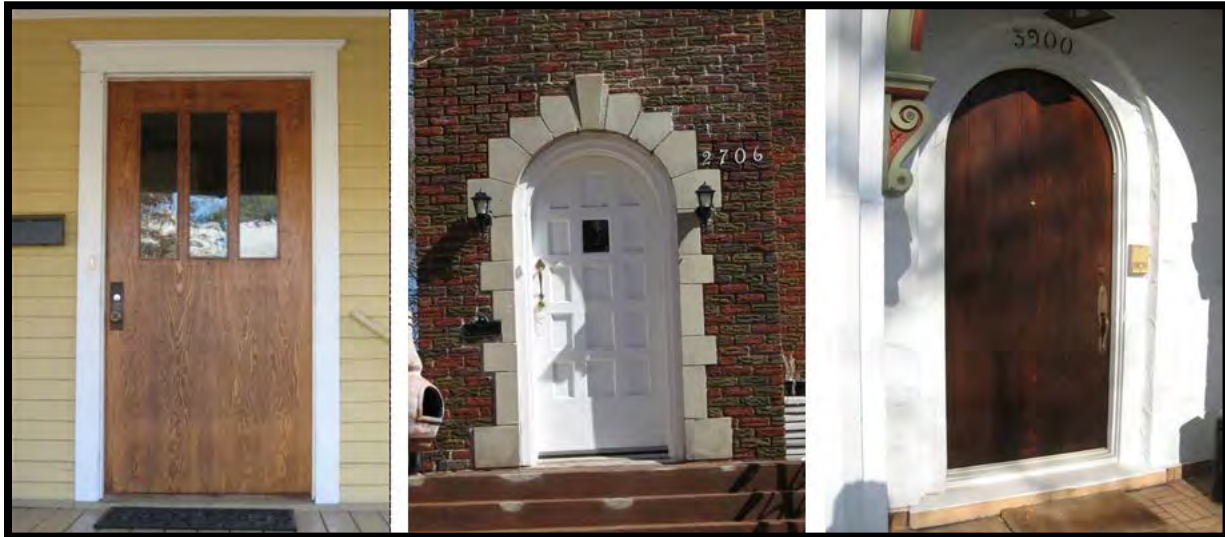
FIGURE 28: CHARACTER-DEFINING DOORS: CRAFTSMAN STYLE, LEFT; ARCHED TUDOR REVIVAL STYLE, CENTER; ARCHED SPANISH COLONIAL REVIVAL STYLE, RIGHT.
