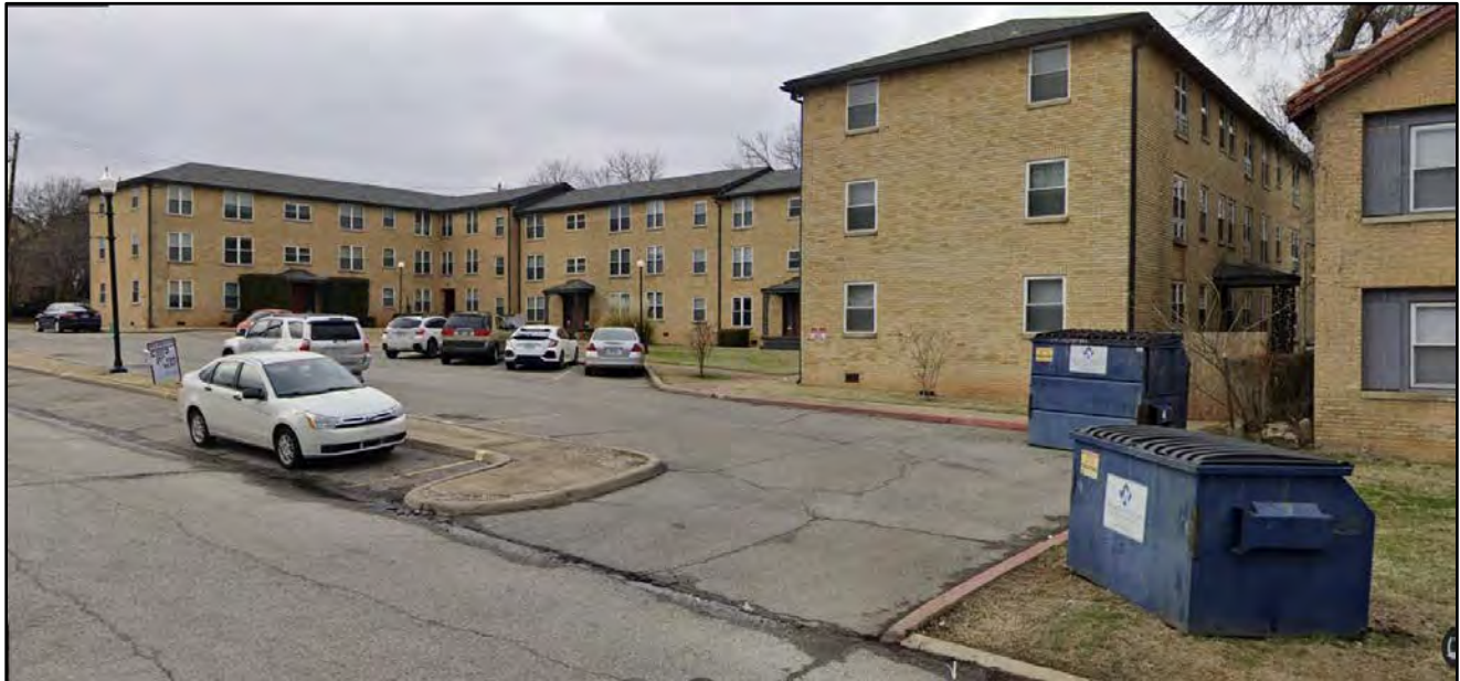
701 Culbertson Drive, South and East Elevations, Looking Northwest, Existing Conditions:
