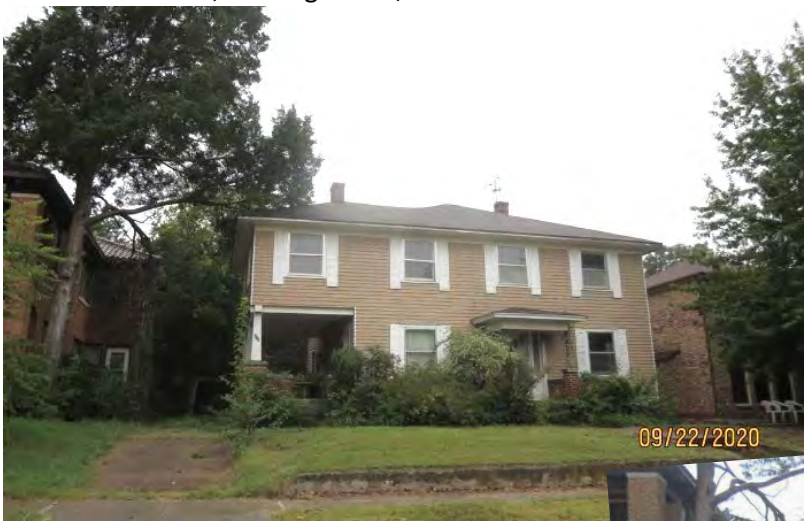
410 NE 16 th Street, Existing Home, North Elevation:
