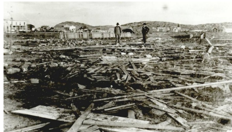
Tornado damage at Snyder, Oklahoma Territory, May 1905
