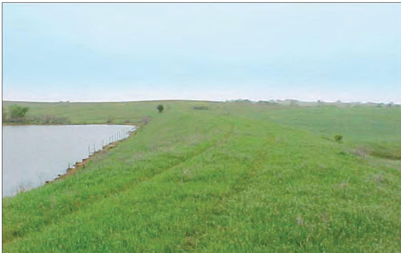
Figure 2: A properly maintained dam using short grasses without trees or shrubs
