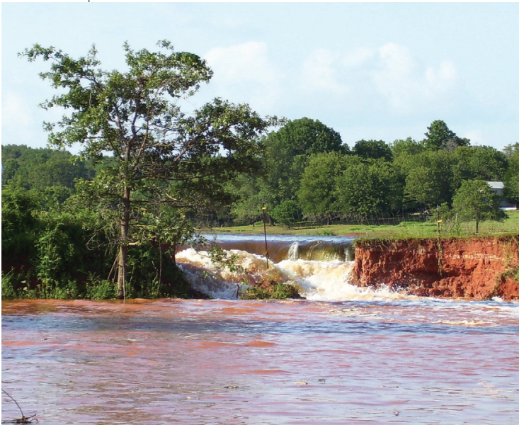
FIGURE 3.1 EMBANKMENT DAM FAILURE IN CLEVELAND COUNTY
